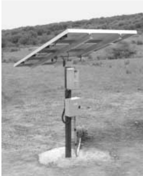
Setting an array pole in concrete.
