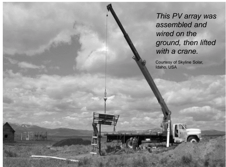
Setting an array pole in concrete.
