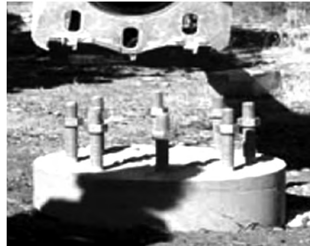
A typical pier foundation ►
