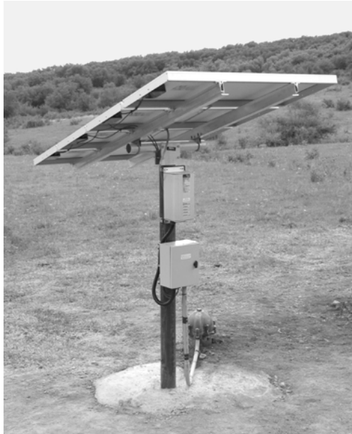
Setting an array pole in concrete.
