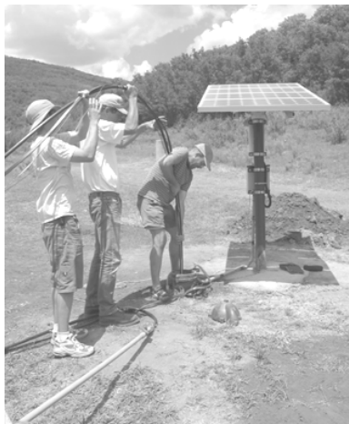
PV array assembly. The mounting pole is short enough to facilitate assembly without mechanical assistance.
