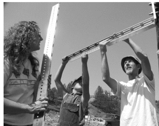
PV array assembly. The mounting pole is short enough to facilitate assembly without mechanical assistance.
