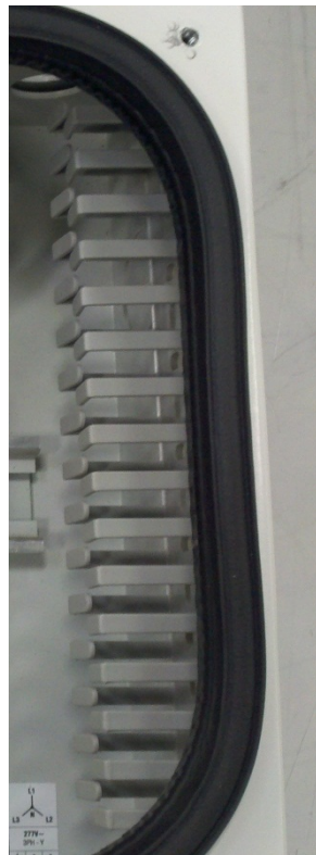
Front switch – cable guides
