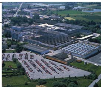
Stiebel Eltron's plant in Holzminden, Germany.
