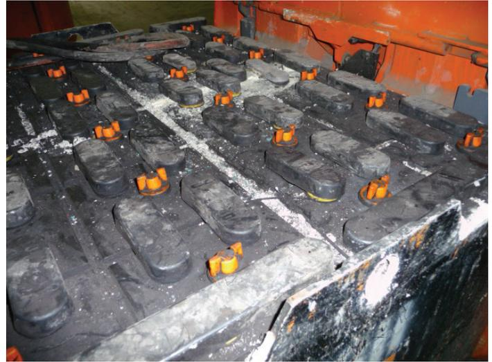
Figure 2: Example of lead acid battery corrosion
