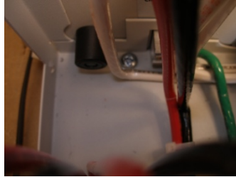
Chassis ground connection to inverter
