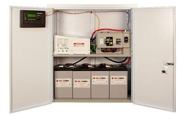
As seen above the very Left battery has its Negative terminal to the Left. The series string continues across to the very right battery where the positive terminal is on the far right. The illustration below shows how to wire the 4 batteries.
