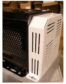
If the E-Panel kit was supplied with a DC end cover, install it using two  $10-32 \times 5/16$ " taptite screws.
