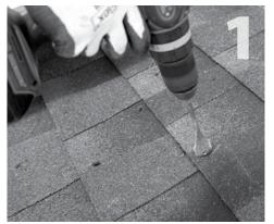
Mark center of rafter. Using the flashing as a template, mark the drill point so the flashing reaches up into the 3rd shingle course. Drill your conduit hole next to the rafter so you can secure the conduit below the roof surface (see Drawing 2). For 1/2" conduit, drill 7/8" hole; for 3/4" conduit, drill 1" hole; for 1" conduit, drill 1-1/4" hole.
