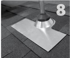
Slide collar over the conduit all the way down to the flashing.
