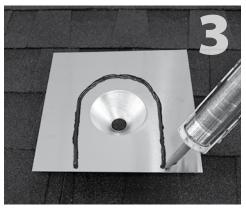
Apply sealant compatible with the roofing material on the underside of the flashing in an upside down U.
