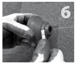
Cut EPDM collar (item 2) to appropriate conduit size (see Drawing 1, Detail A on reverse). Take care to cut a clean, level line.
