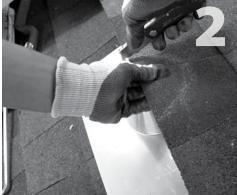
Slide flashing (item 1) into position centering the flashing hole with drilled hole. Remove any nails that prevent getting the flashing into position. Using a hook blade, cut shingle around cone to allow correct placement of flashing. Flashing should not hang over bottom (drip) edge of shingle below.
